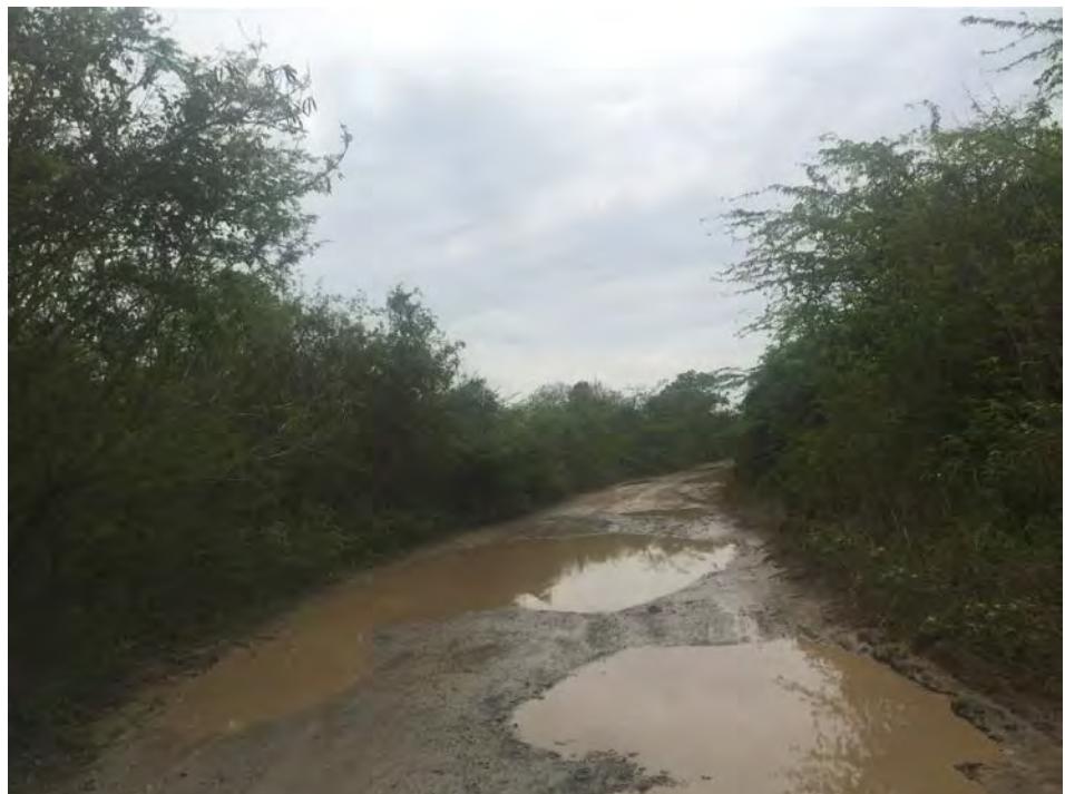
Photo 4. Larger water and sediment deposits on the access road area just before the start of the remedied section of the road.
