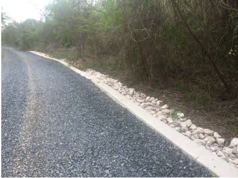
Photo 5. Beginning of access road green infrastructure sediment and erosion control.
