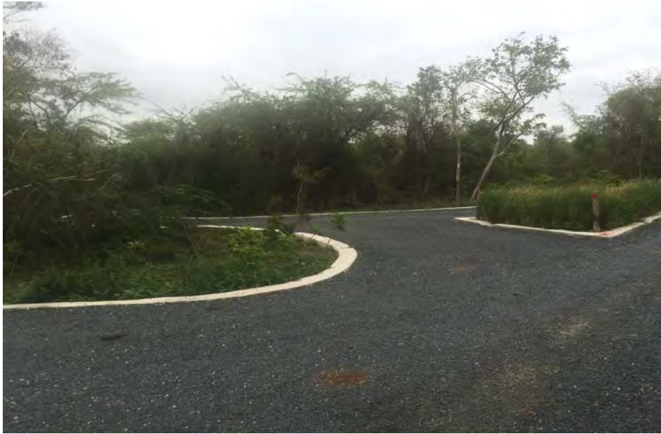
Photo 8. Turnaround area with rain gardens. With the exception of some small plants the vegetation appeared to receive little to no damage.
