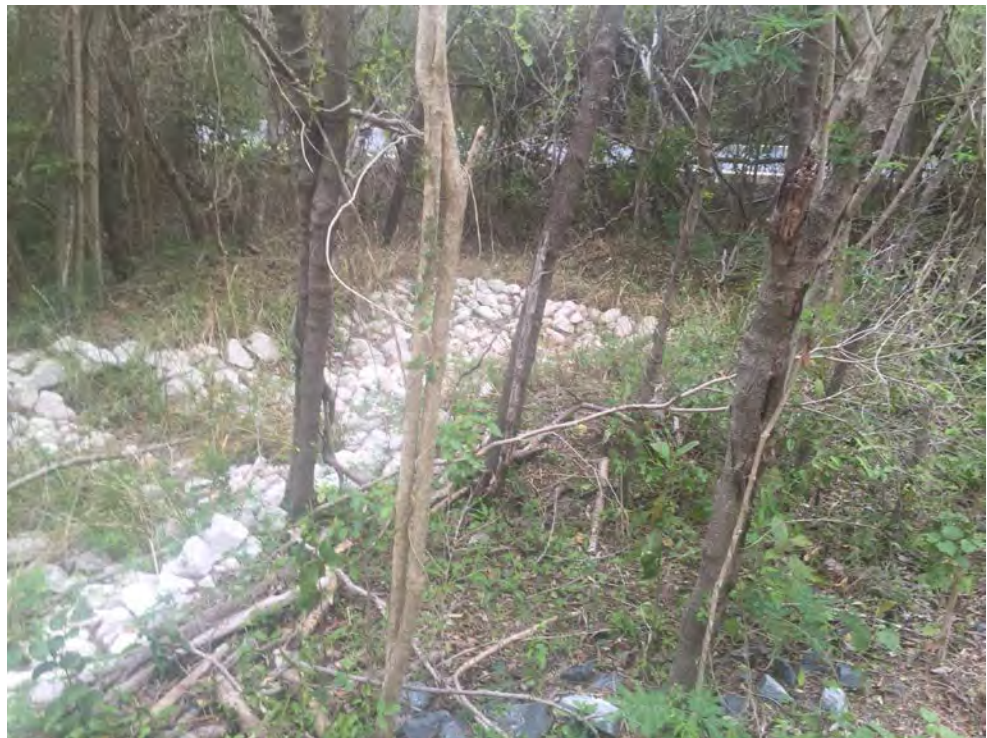
Photo 6. Vegetated sediment trap on connecting road to Panteón beach; it was free of sediment which demonstrates it is working properly.
