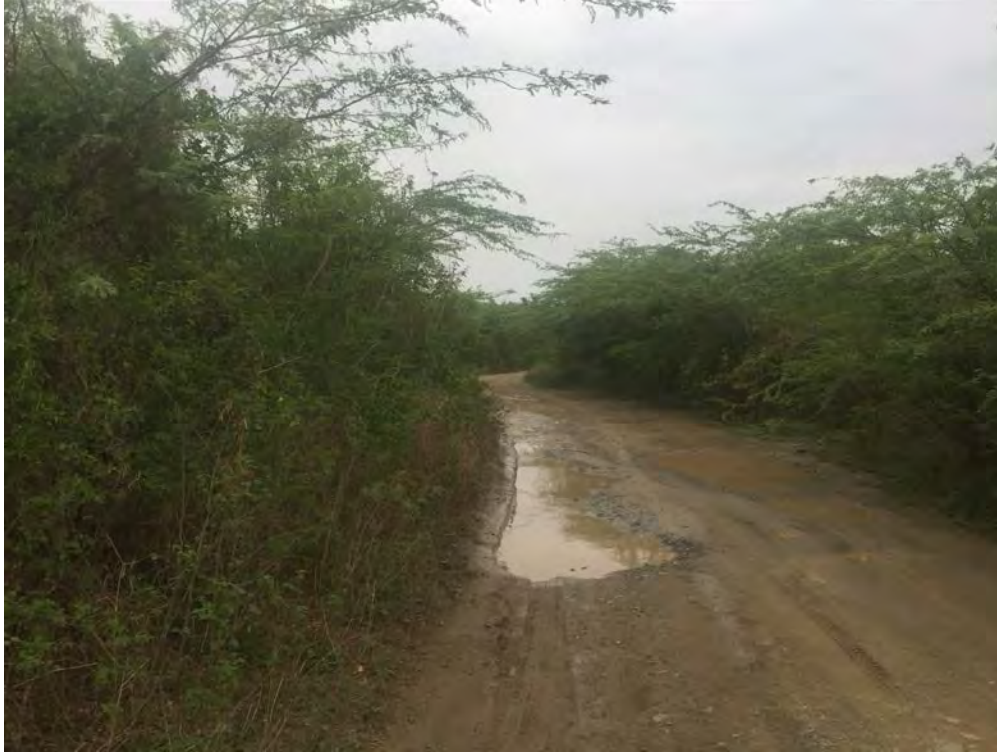
Photo 3. Puddles and deposited sediment on the road.
