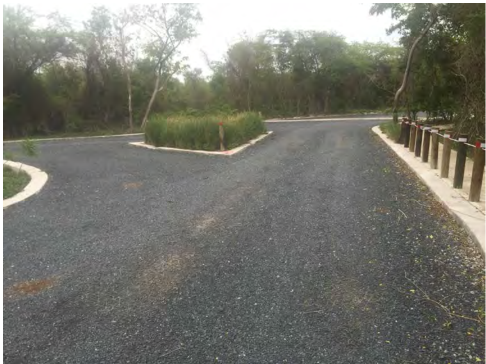
Photo 7. Remedied road to the Bay with permeable pavement and rain gardens to the sides and center. The area was dry and showed no signs of damage.
